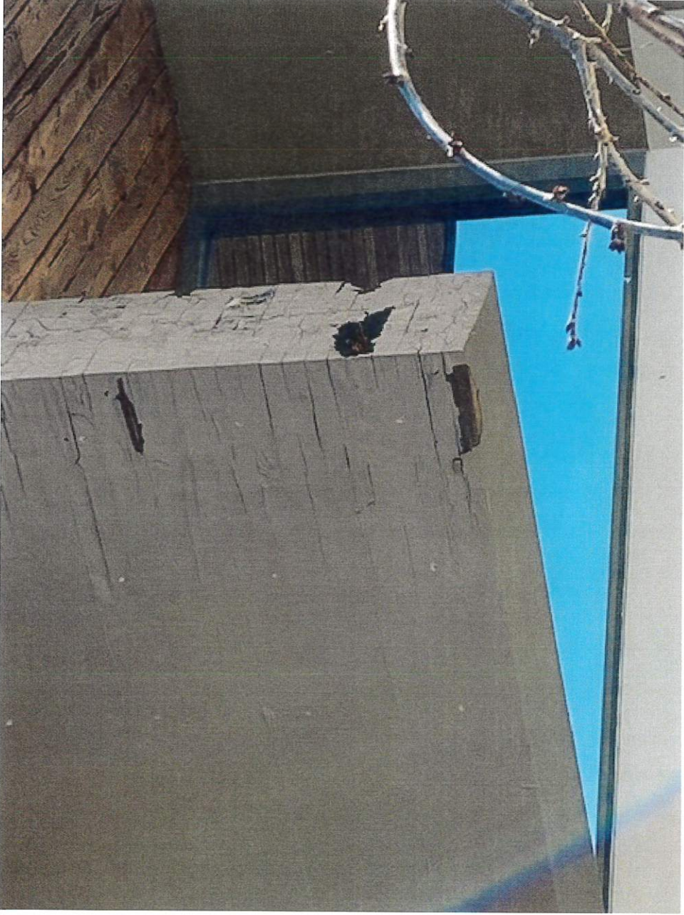
Beams on outside of Plymouth Cultural Center
