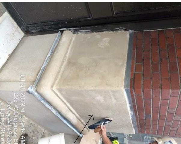
Second Coat Application of Stone Product
