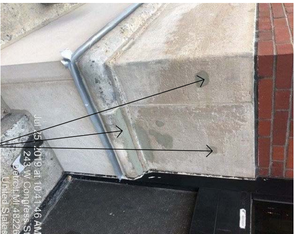
Damaged Locations Repaired With Stone Patching Product
