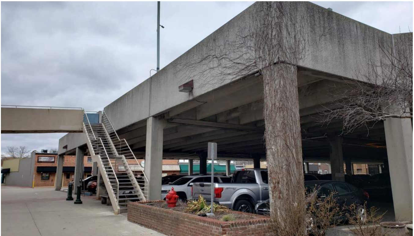
Pedestrian bridge and steel stair at east elevation of parking structure
