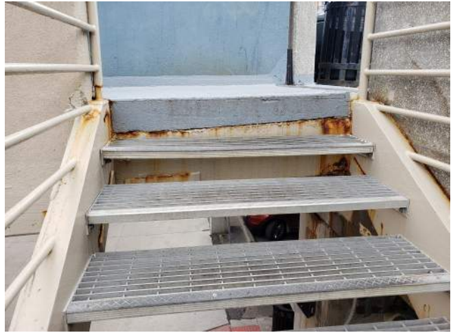
Existing stair/pedestrian bridge connection
