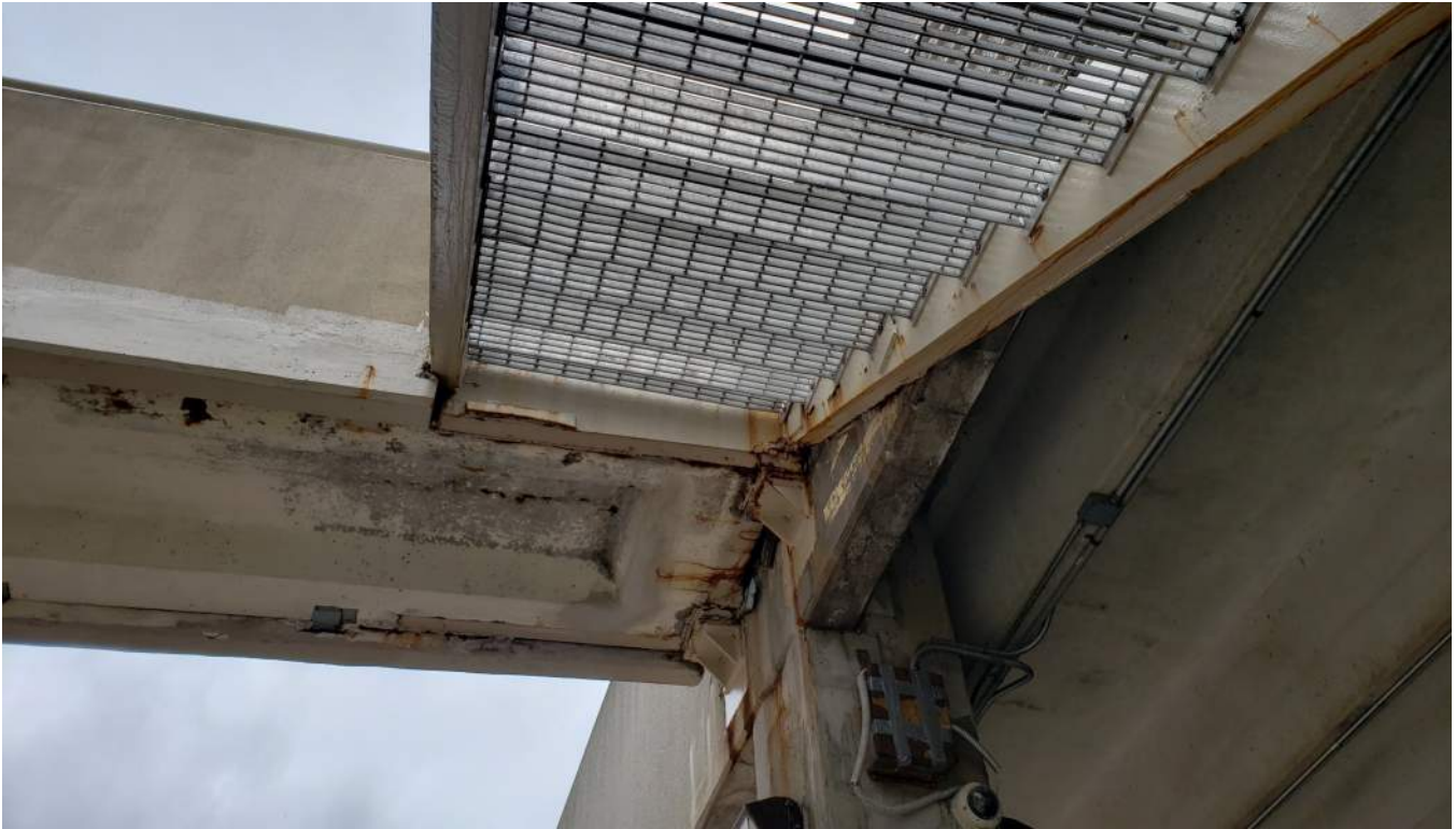
Existing stair-to-bridge and bridge-to-structure precast connections
