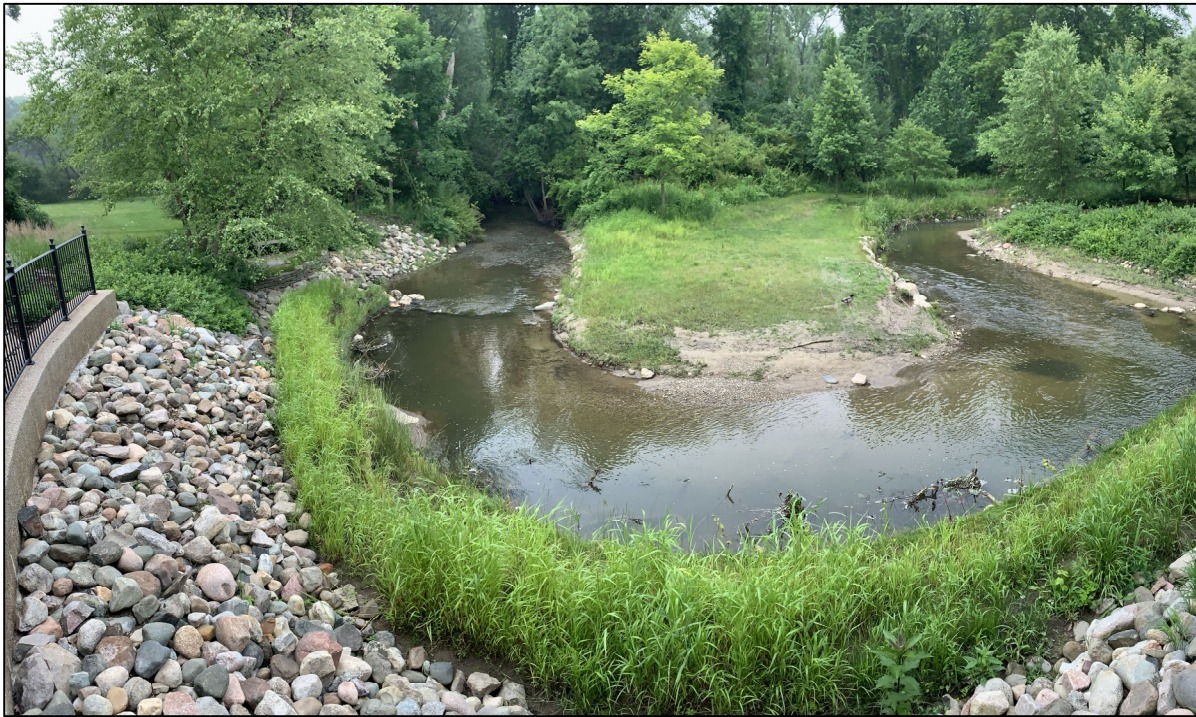
Figure 2. Example Brush Toe Stabilization, Fabric-Encapsulated Soil Lift and Native Seed
